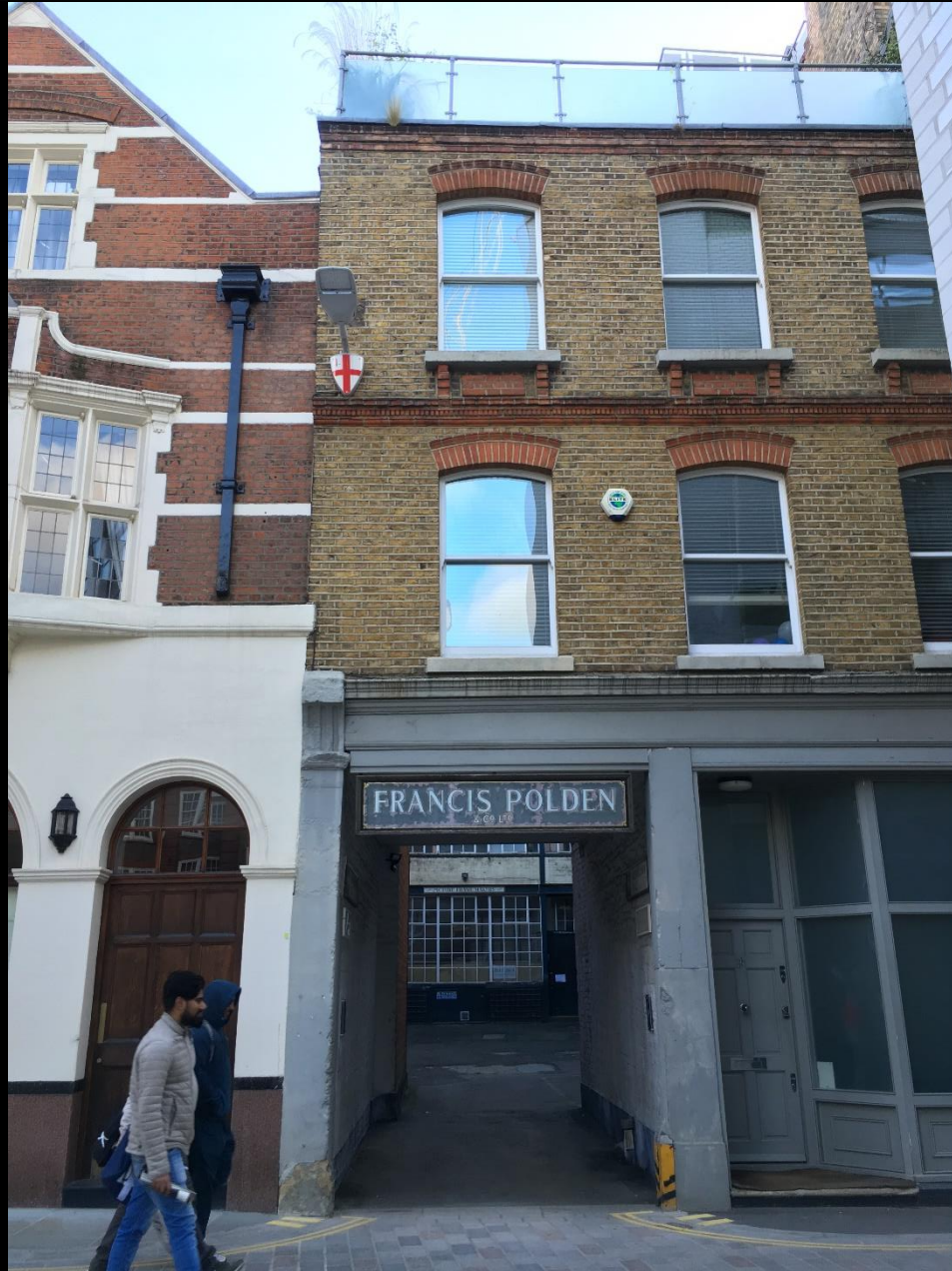
Existing front view
