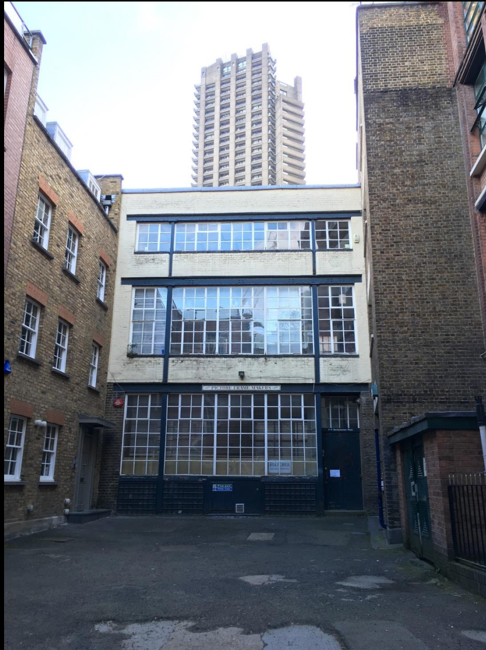
Existing courtyard view
